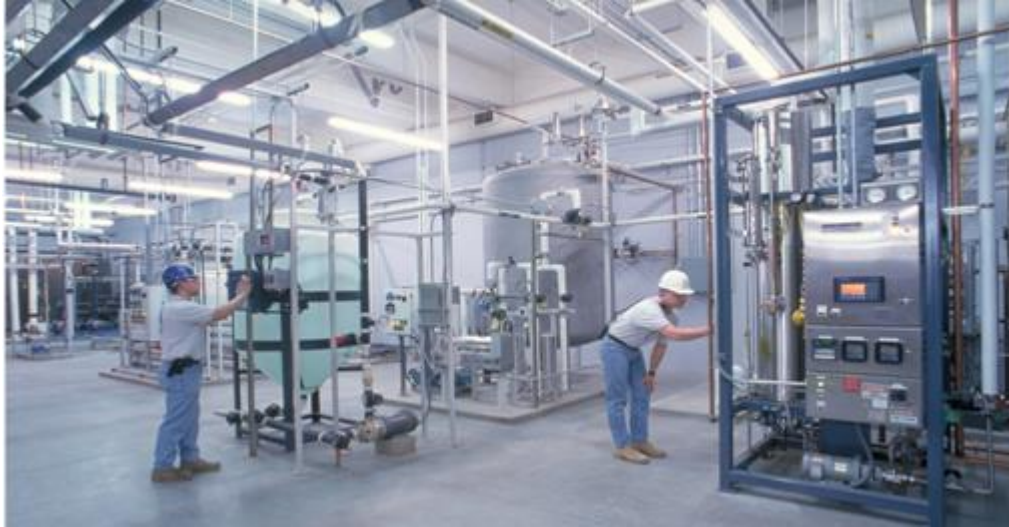
Figure 1-15. Facilities and Metrology technicians
