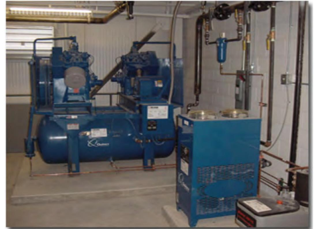
*Industrial air compressor with a refrigeration drier*
