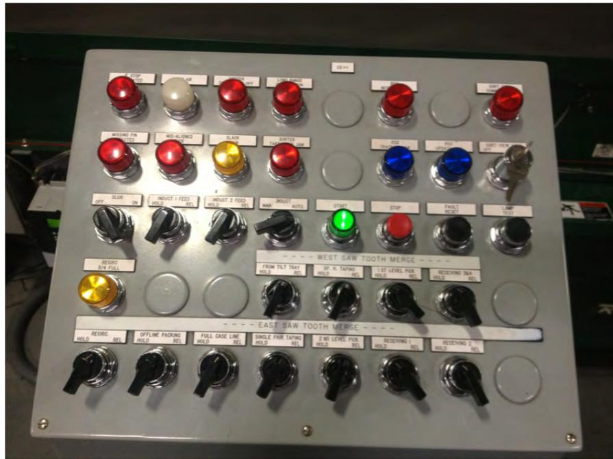
*Operators' Control Station which can be used for manually switching and overriding PLC's Inputs or Outputs for operations indicated by illuminated lights*
