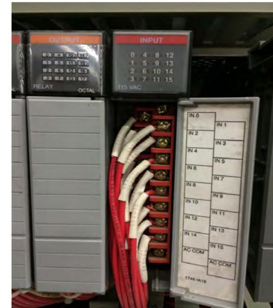
*PLC input board with wire markings beginning with 1 and followed by the circuit number*
