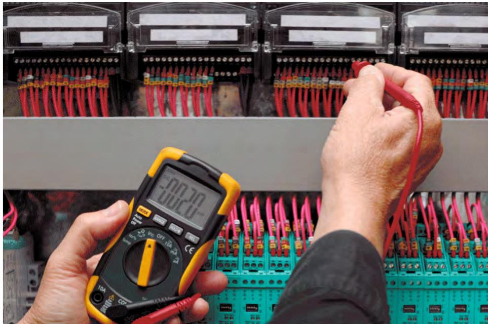
*Electrical testing of low voltage control circuits*
