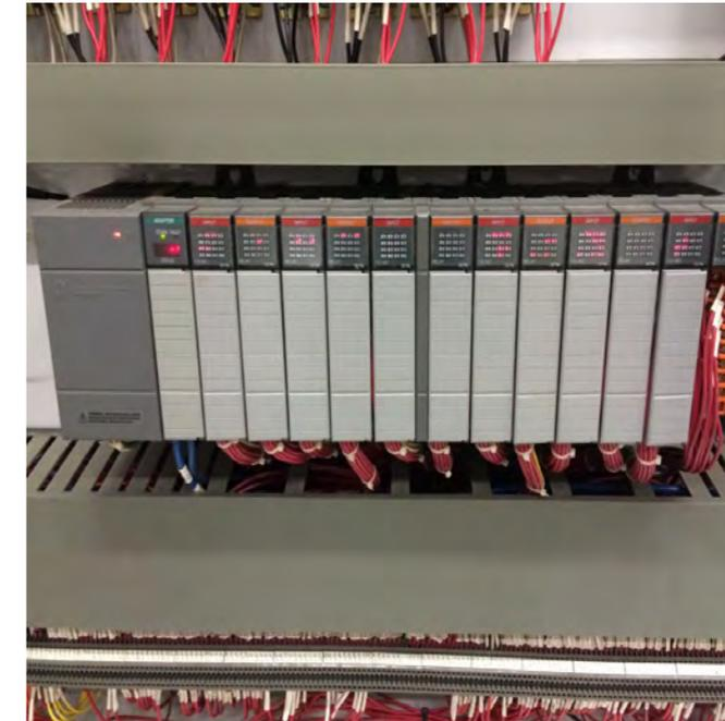
*PLC rack of input and output boards*
