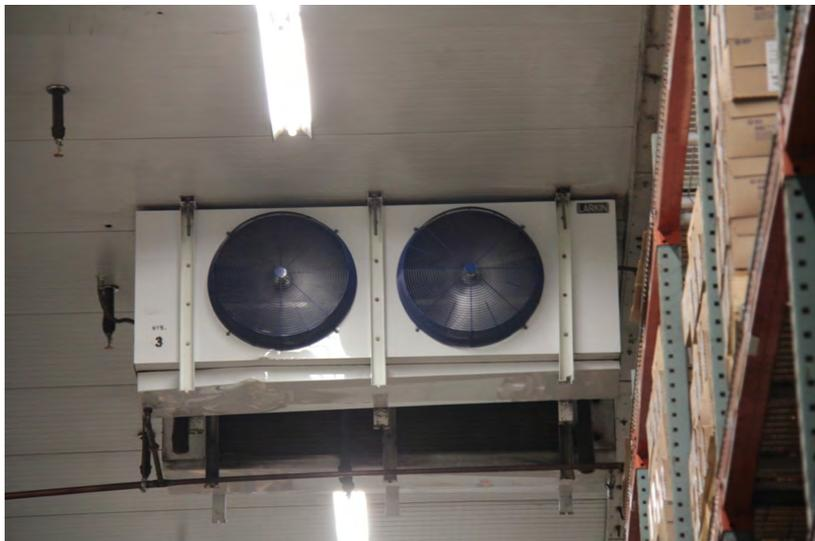
*Evaporators for a commercial refrigerator*
