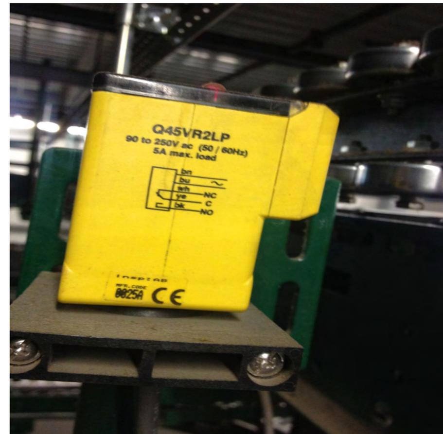
*Photo Eye 120 Volt input to PLC input modules*
