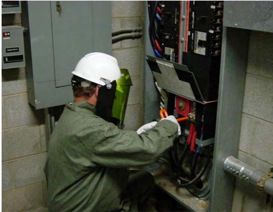
*Protective clothing worn during electrical testing on a live circuit*
