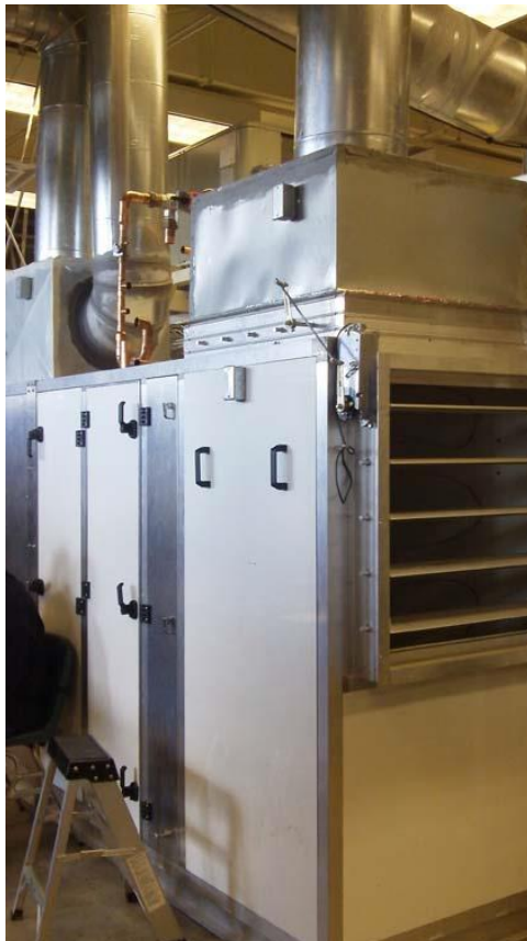
FIGURE 1 - Economizer on built-up AHU in lab. Controls fully accessible for adjustment, setting up faults, or commissioning activities.
