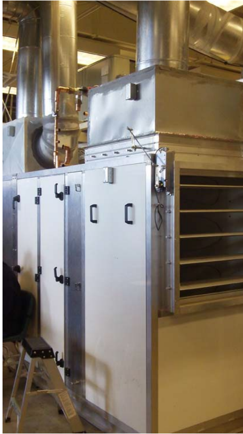
FIGURE 1 - Economizer on build-up AHU in lab. Controls fully accessible for adjustment, setting up faults, or commissioning activities.
