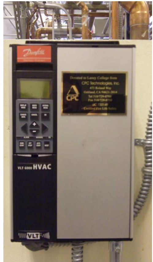
FIGURE 2 - Variable Frequency Drive, 3 are connected to water circulation pumps in lab. Can be programmed by students, faults can be set up by instructor.
