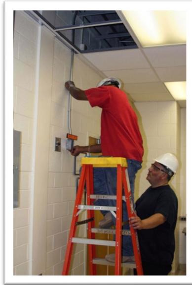
Pictures of BAS students working in C-building, mounting conduit & sensors, running network cabling & commissioning control systems
