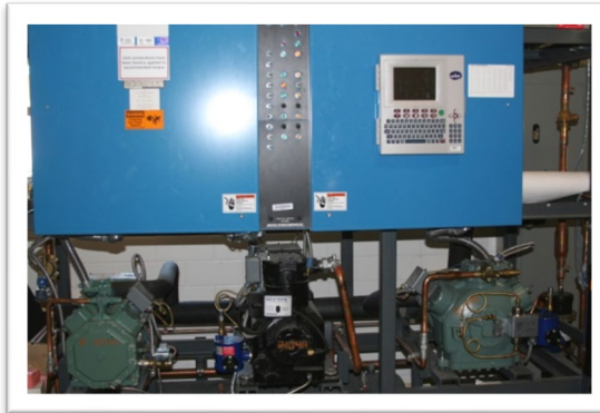
Hill Phoenix Rack system with 3 compressors & CPC controls
