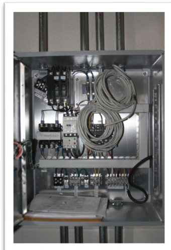
Samples of student-mounted controls, conduit & cabling (BUAS 2030)
