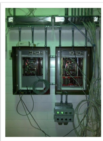
Samples of student-mounted controls, conduit & cabling (BUAS 2030)
