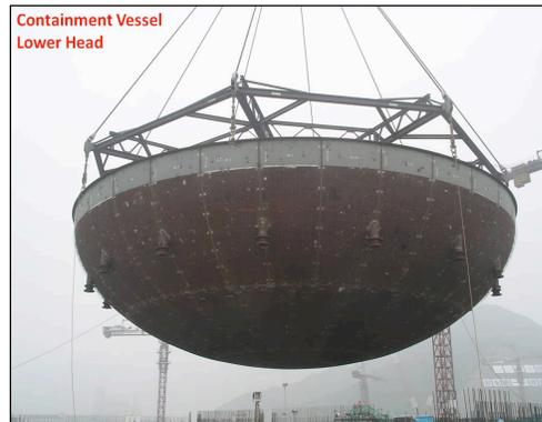
This picture was taken in 2010 at the Sanmen AP1000 site in China. The CV bottom head is being lowered into place on the Nuclear Island.
