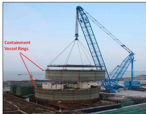
This picture was taken in 2010 at the Sanmen AP1000 site in China. The Crane is lowering the 2nd CV ring into place.
